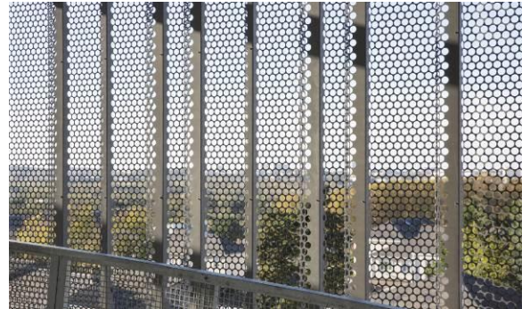
CAR PARK IN SAINT LAUD, ANGERS, FRANCE ZINC SHEETS - QUARTZ-ZINC® ARCHITECTURE FIRM: AZÉMA ARCHITECTES PHOTO CREDIT: PAUL KOZLOWSKI
