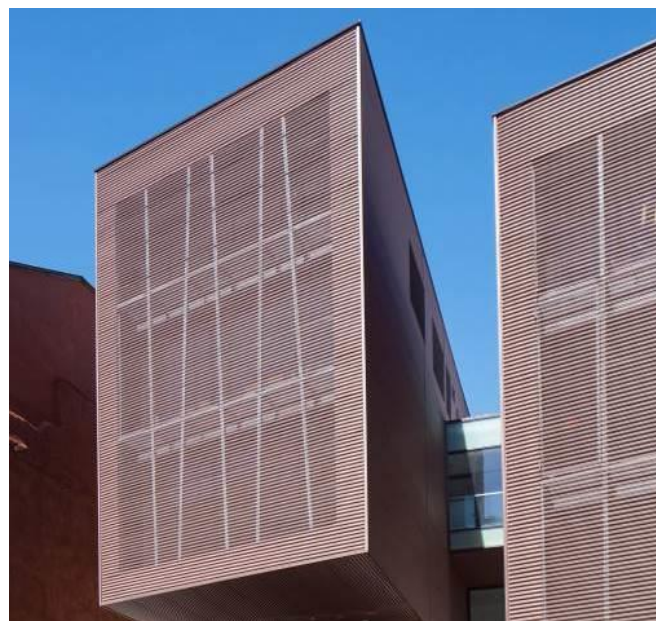
MUNICIPAL TRAINING AND EMPLOYMENT CENTRE IN RODEZ, FRANCE VMZ PERFORATED SINE WAVE PROFILE - PIGMENTO® RED ARCHITECTURE FIRM: LACOMBE DE FLORINIER PHOTO CREDIT: PAUL KOZLOWSKI + GILLES TORDJEMAN
