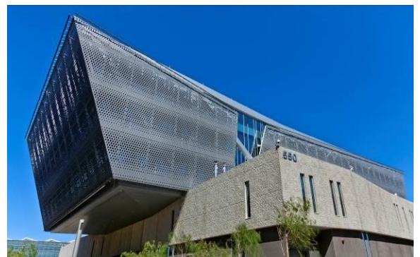
POLICE HEADQUARTERS IN PHOENIX, USA VMZ PERFORATED COMPOSITE - QUARTZ-ZINC® ARCHITECTURE FIRM: GABOR LORANT ARCHITECTS PHOTO CREDIT: GILBERTSON PHOTOGRAPHY
