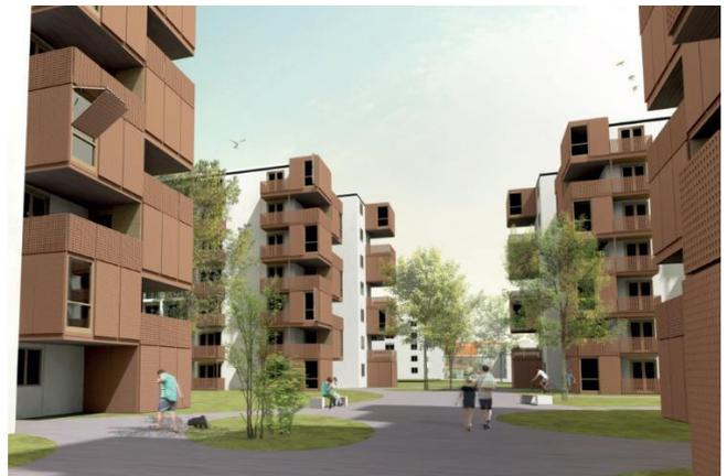
Work on an occupied site required precise construction drawings in order to minimise the construction time. The extensions are made of prefabricated independent modules. The insulated, waterproof interlocking boxes are attached to the existing structure through a process that reduces installation time and related pollution (noise, dust, etc.). The students involved the residents from the outset in order to mitigate their fears and provide an appropriate response based on each person's needs.
